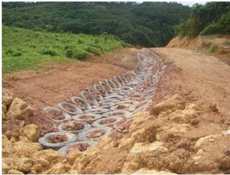
Figure 3. The drainage system constructed and reinforced with stone or other materials to reinforce the drain base.
