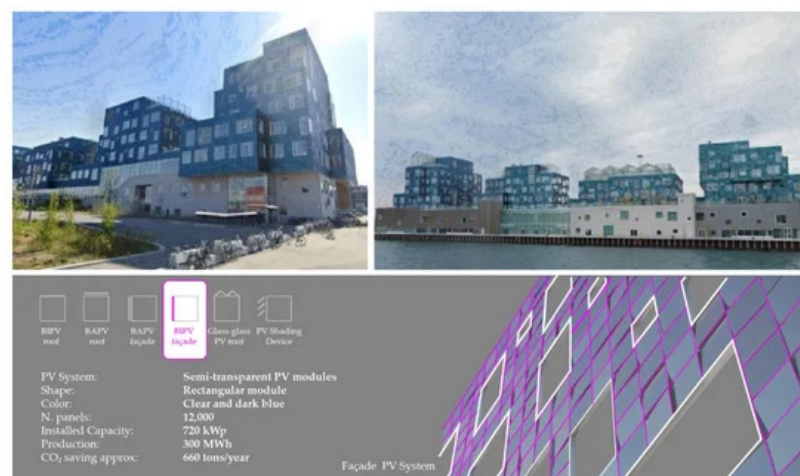
Figure 10. Copenhagen International School (a top view and elevation: Source of illustration Google Earth, Google 2020) (on top). Integration and characteristic of PV systems (on the bottom).
