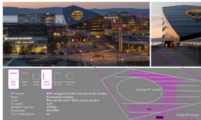
Figure 4. Powerhouse Brattørkaia (photo on top by Ivar Kvaal, with permission from Powerhouse http://powerhouse.no ) (on the top); Integration and characteristics of PV systems (on the bottom).
