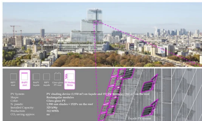
Figure 5. Paris Courthouse east façade (photography with permission of author Sergio Grazia) ( on the top ); Integration and characteristic of PV systems ( on the bottom ).
