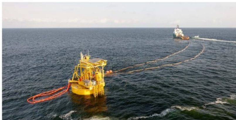
Figure 1. Full replacement operation of floating hoses, submarine hoses, hawsers and a single point mooring (SPM) buoy attached to a service offshore vessel (SOV) by a tug supply boat, located at 35 m water depth in Republic of Congo, Djeno Terminal (Courtesy: Bluewater & South Offshore [24]).
