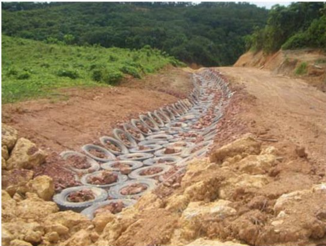
Figure 3. The drainage system constructed and reinforced with stone or other materials to reinforce the drain base.
