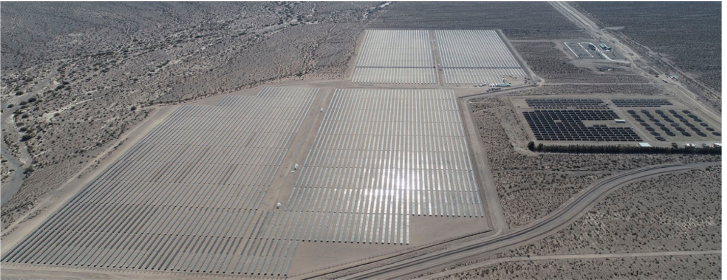
Figure 3. A view of Ullum IV, a 16 MWp photovoltaic plant located in the desertic province of San Juan, which went operative in 2019. Also shown is the San Juan I PV technology testing plant (far right, center).
