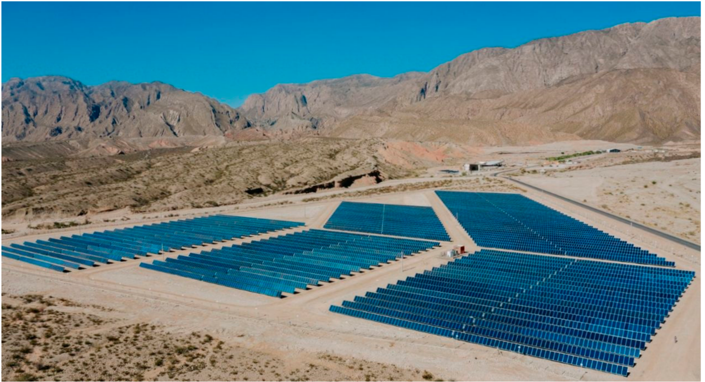
Figure 4. Anchipurac is a small-sized 3 MWp PV solar plant provided by single-axis tracking, located in Argentina's west-central province of San Juan. Photograph courtesy of Estrada.
