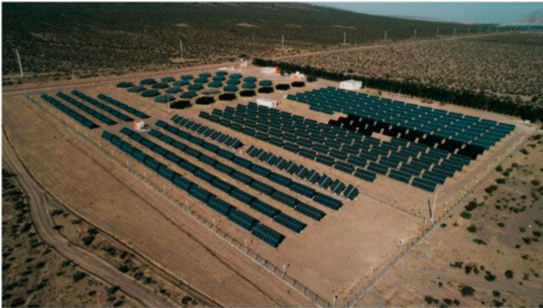
Figure 6. Solar San Juan I pilot solar plant, a 1.2 MW test facility using different module and mounting technologies, including fixed and single axis orientation for crystalline, multicrystalline and amorphous silicon modules. Photograph courtesy of Estrada.
