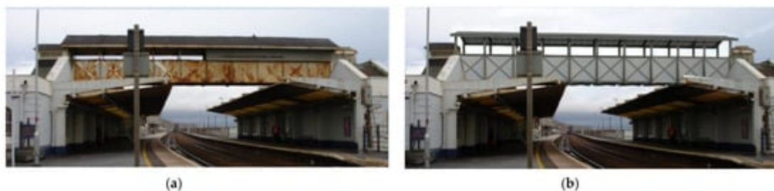
Figure 4. Dawlish pedestrian bridge Exeter UK: (a) Old rusty steel bridge, 1937 [40]; (b) New FRP bridge, 2011 [40].
