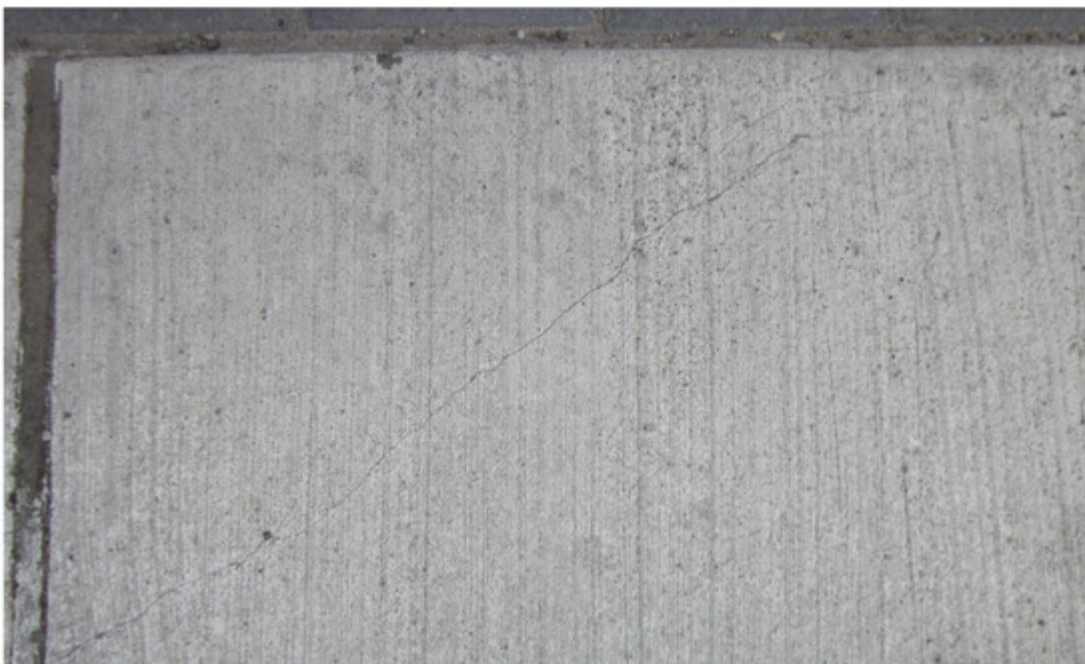
Figure 3. Early-age corner crack in a concrete side-walk slab; this crack appeared within 35 days after concrete placement; the concrete slab was cured by curing compound.
