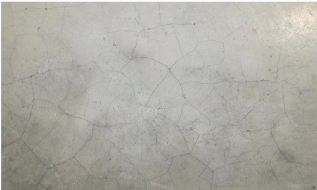
Figure 5. Early-age map cracks that occurred in a newly cast concrete floor slab; these cracks appeared within 14 days of concrete placement; the floor slab was cured by spraying of water.
