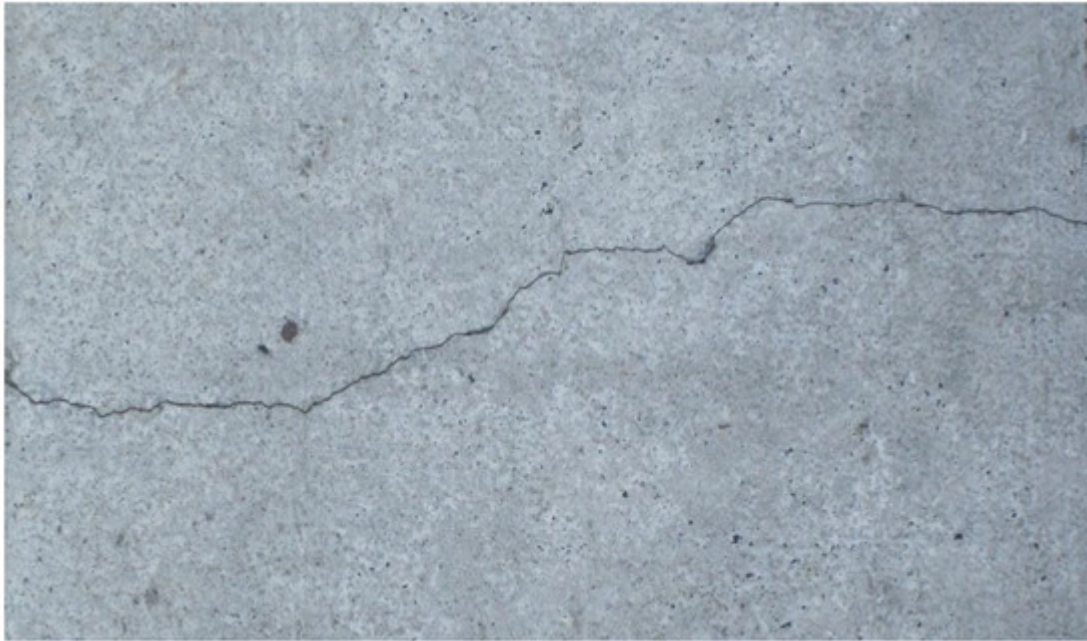
Figure 6. Restrained shrinkage cracking that occurred in a roadside concrete curb; this crack initiated within 56 days of concrete placement; the curb was cured with curing compound.
