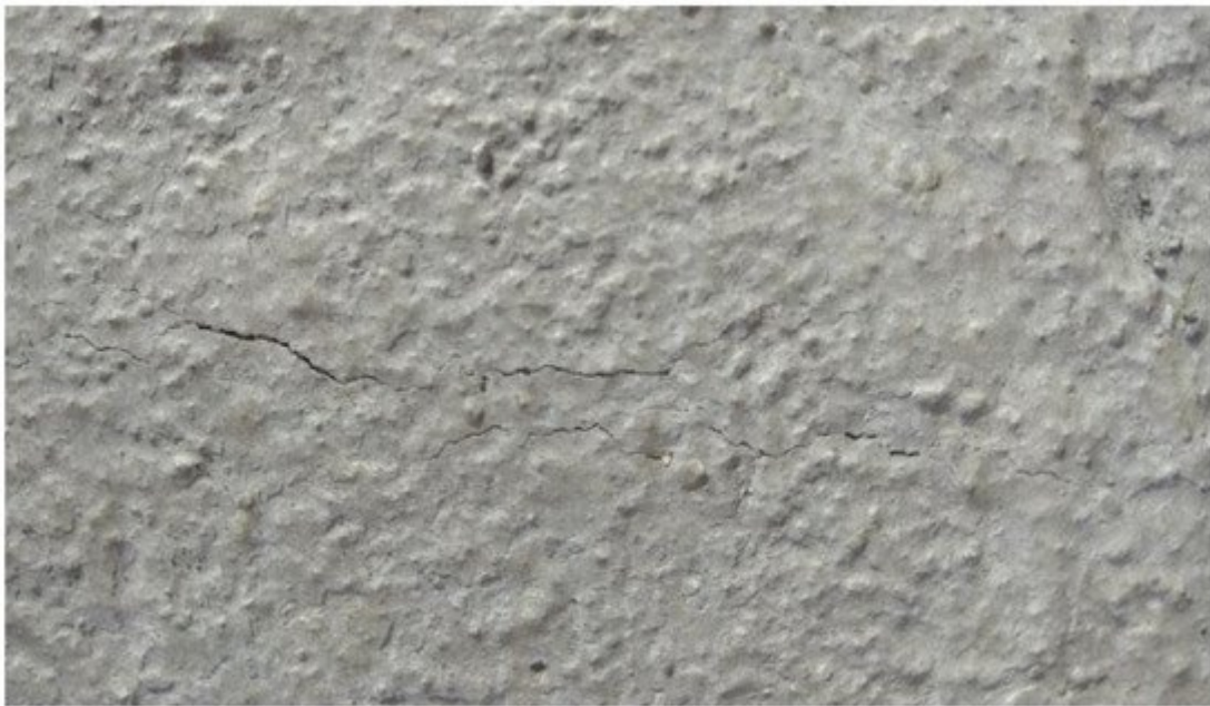
Figure 1. Early-age transverse cracks that occurred in a newly cast reinforced concrete column; these cracks occurred within three days after placing of concrete; the column was cured by wet burlap.
