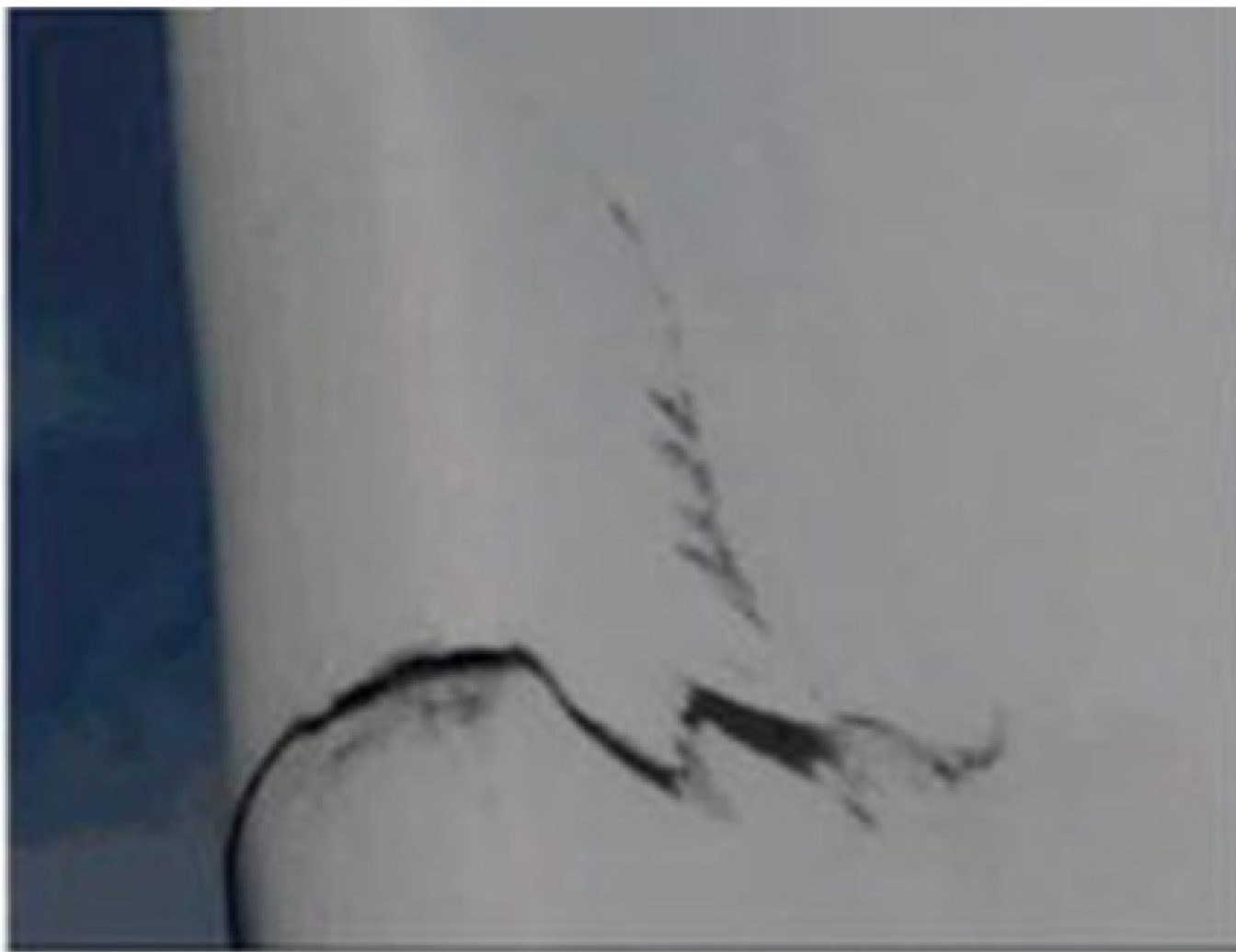
Figure 2. Transverse cracks found on the trailing edge of a wind turbine blade.
