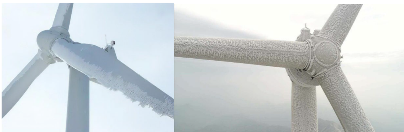
Figure 6. Ice on wind turbine blades.
