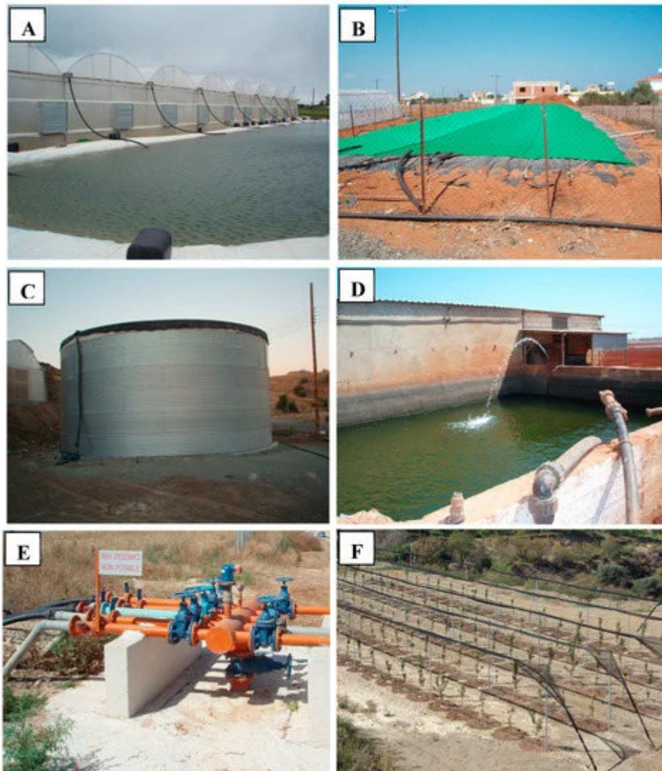
Figure 4. Rain water harvesting and storage in open reservoir (A); water storage in a covered reservoir minimizing water evaporation losses and algae growth (B); a commercial closed water reservoir (C); blended water from different sources (D); a water supply main manifold of recycle water (E); localized irrigation and net protection in a tree cropping system (F).
