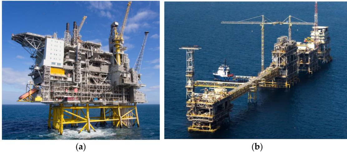
**Figure 1.** Typical platforms showing (a) conventional jacket platforms and (b) bridged fixed jacket platform on Zuluf oil field in Arabian Gulf, offshore northeast Saudi Arabian coast, with the water depth of about 40 m (Image (b) Courtesy: Saudi Aramco).
