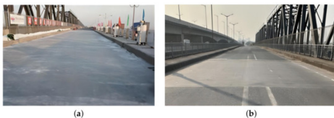
Figure 7. Mafang Bridge using steel-UHPC composite deck: (a) Under construction; (b) After 12 years in service.
