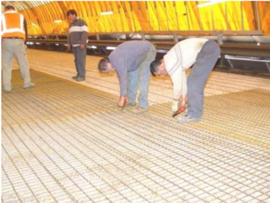
Figure 6. Deck replacement of Galand Bridge using glued UHPC layer.
