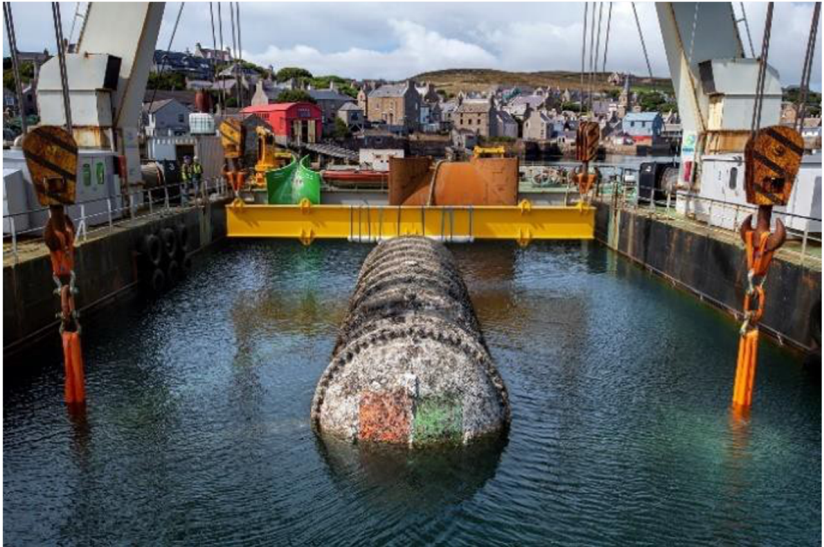
Figure 7. Retrieval of Microsoft's Northern Isles data center (Project Natick) in July 2020.
