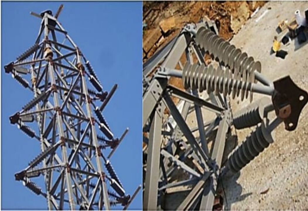
Figure 15. Composite cross-arm insulators (four pultruded structure components) [43].
