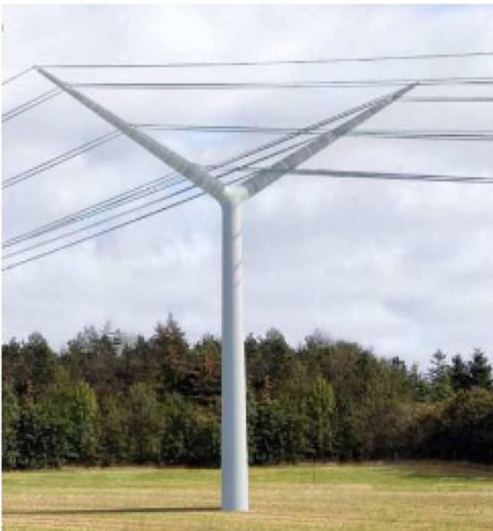
Figure 20. Y-shaped composite pylon overhead line tower [57] .
