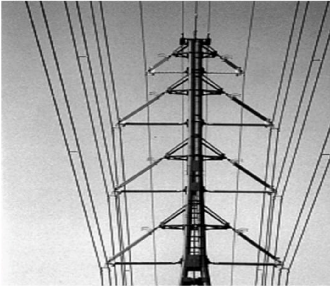
Figure 3. Front view of the compact tower [11] .
