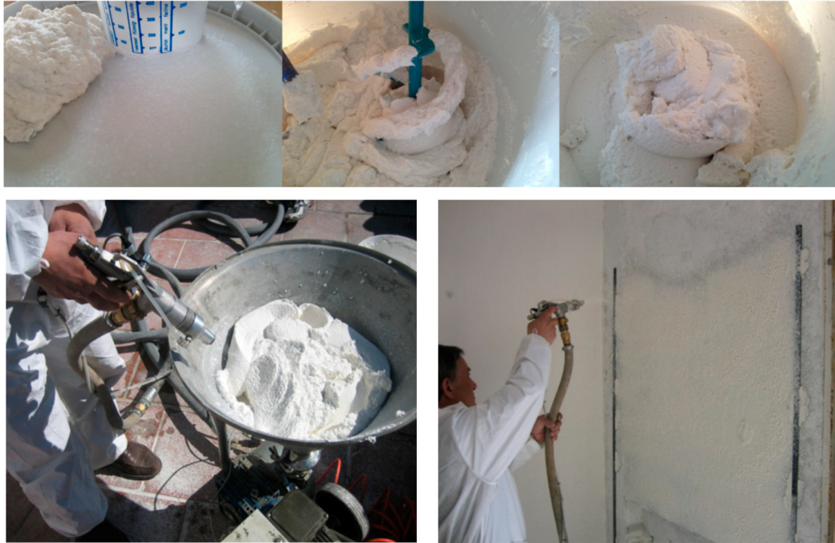
Figure 6. Aerogel-based plaster in building constructions [27].
