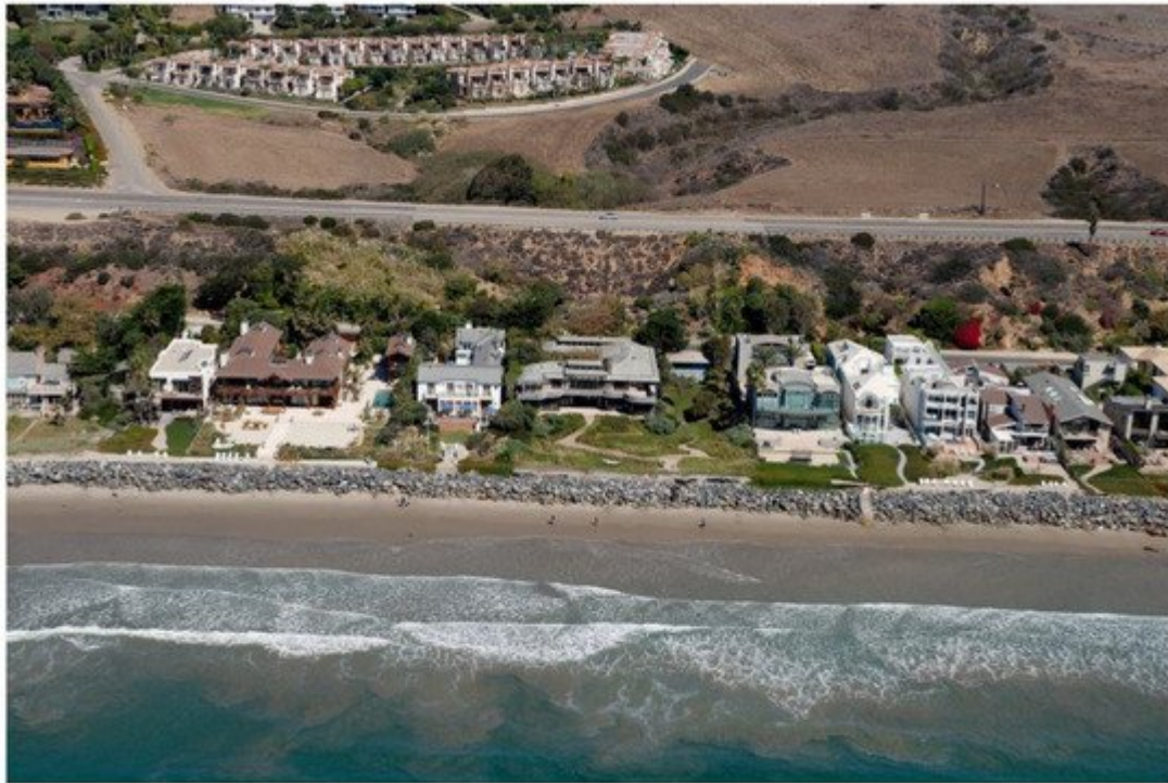
Figure 5. Rip-rap revetment armoring a section of the Malibu, California (USA) shoreline. Courtesy: California Coastal Records Project.
