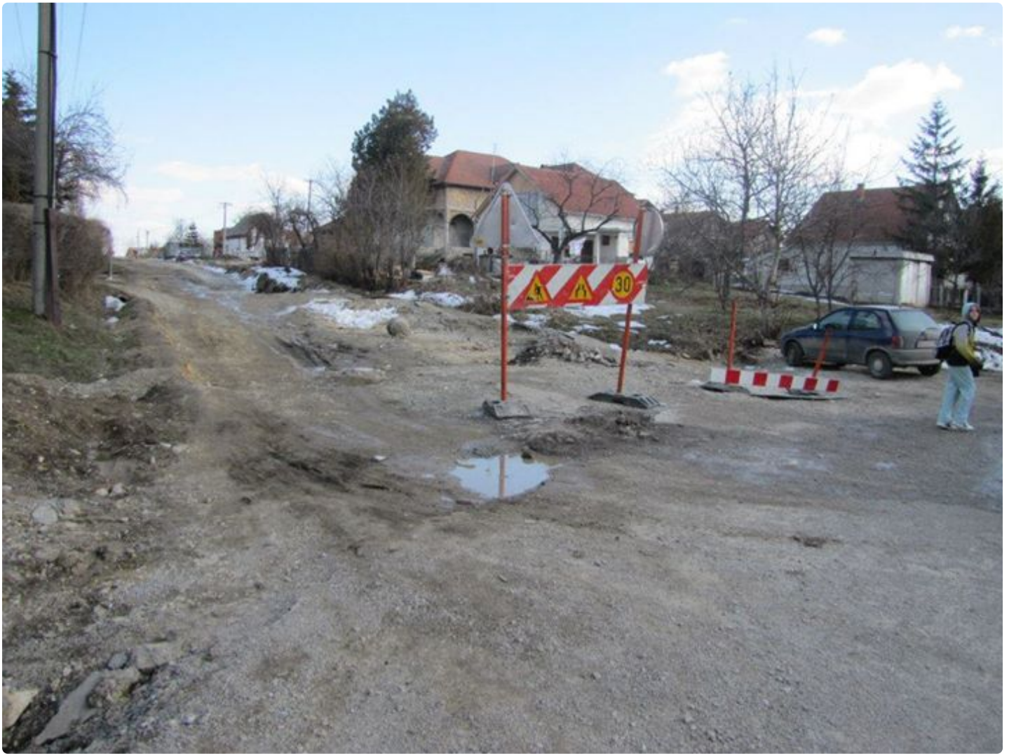
Figure 1. An example of poor regulation and direction of traffic in the roadwork zone.
