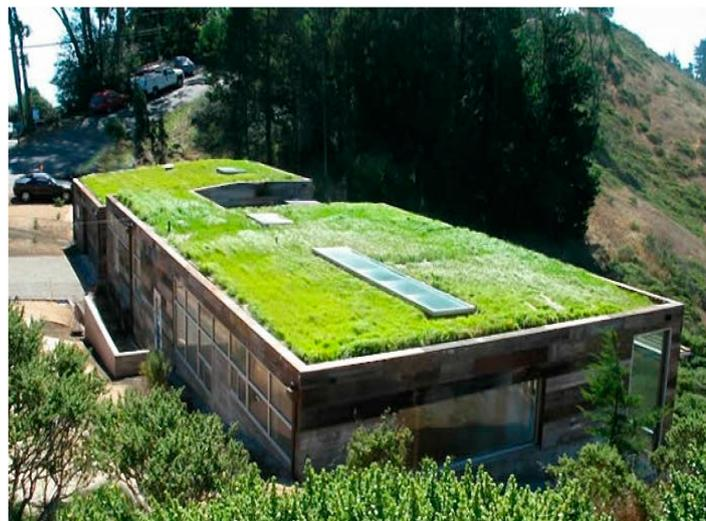
**Figure 5.** Extensive green roof [17].
