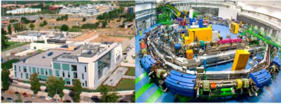
Figure 2. Left: in front the Centre for Oncological Hadron therapy (CNAO) hospital building, in the back the power station and the roof of the synchrotron vault. Right: view of the synchrotron and of the beam transport lines.
