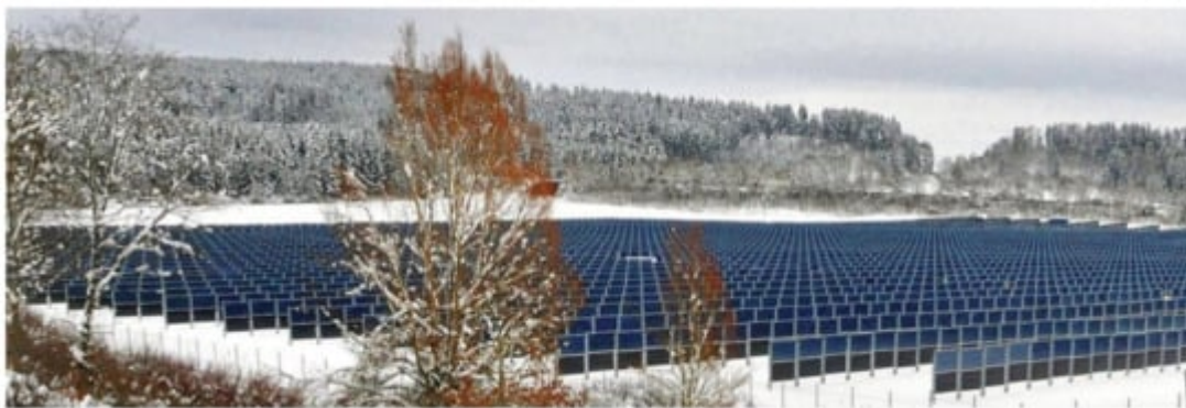
Figure 8. Vertical bifacial PV system by Next2Sun in winter, showing one of the advantages not being covered by snow [8] .
