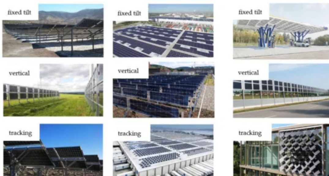
Figure 5. Possible bifacial installations for utility scale (left), flat roof-top (middle) and integrated (right).
