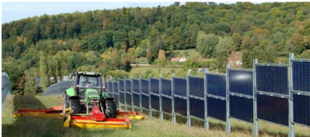
Figure 7. Vertical bifacial PV system by Next2Sun showing the advantage of double use of land [8] .
