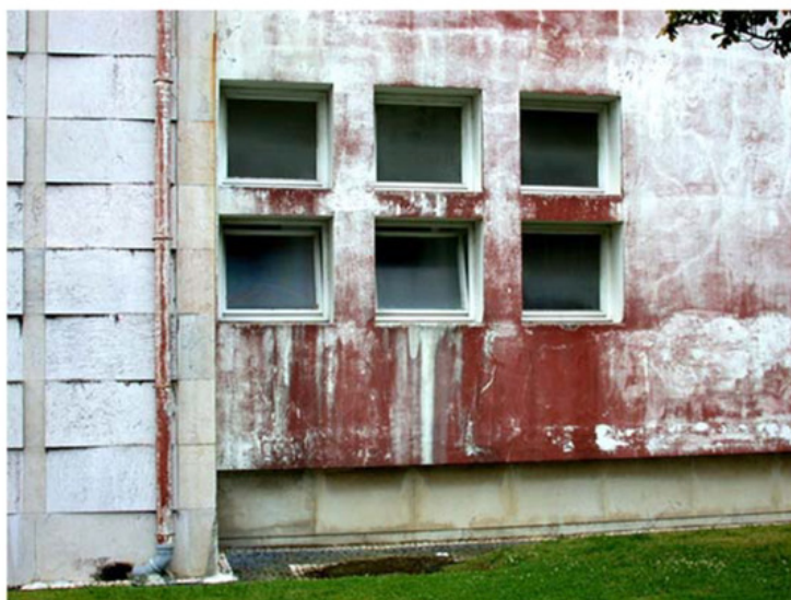
Figure 4. Trentepohlia algae forming deep red discoloration on the painted wall of a public building in Ponta Delgada, Azores, Portugal.
