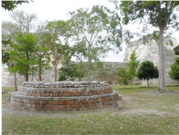
Figure 5. Stone altar in the architectural zone of Becan, Campeche state, Mexico, showing red staining ( Trentepohlia ) on North and East facing sides.
