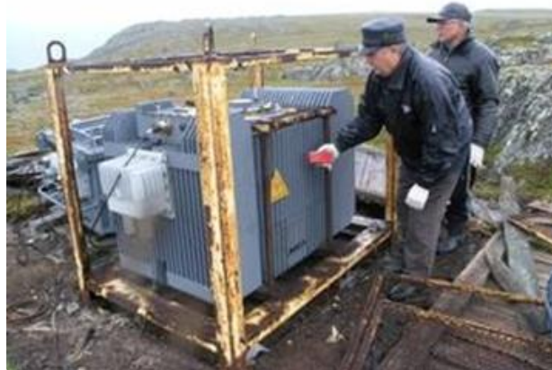
Figure 3. RTG used to supply power to lighthouses and navigation beacons [19]
