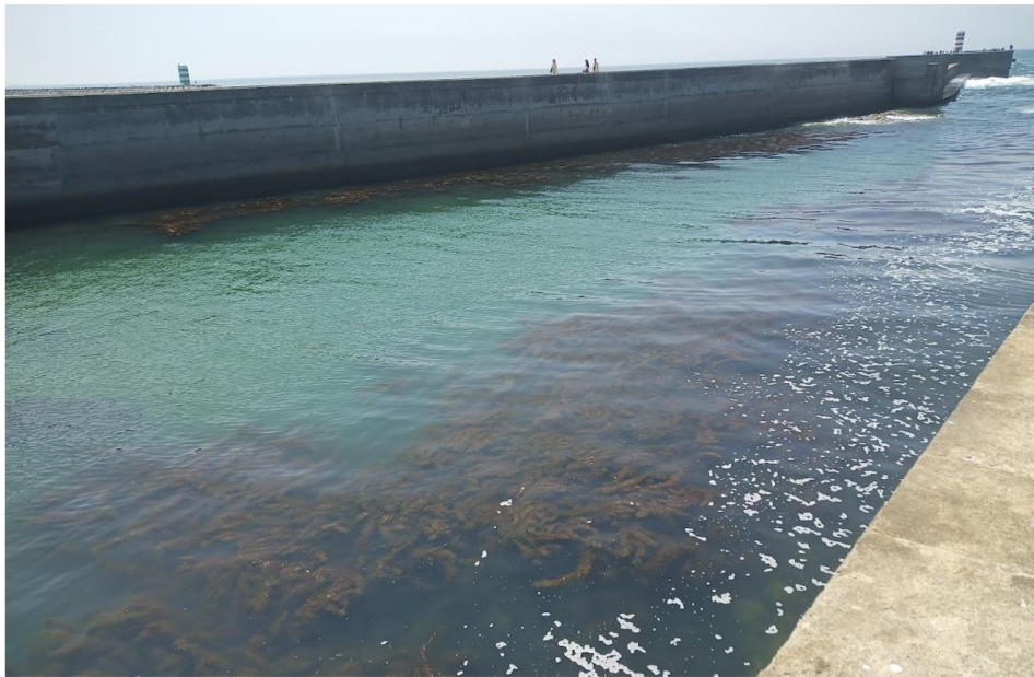
Figure 3. Seaweed beds on aquatic habitat reducing the wave effect in coastal shore, trapping the sedimentation and reducing coastal erosion.
