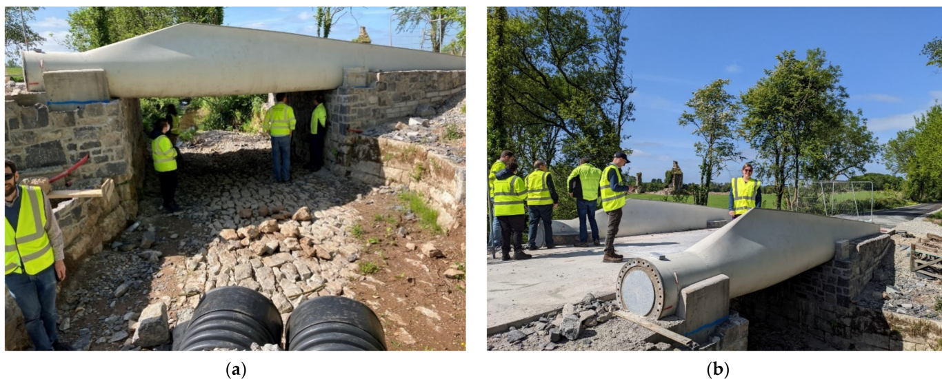
Figure 4. Re-Wind Network's first footbridge in Cork, Ireland, constructed from decommissioned wind turbine blades in January 2022: (a) Front view of the blade bridge; (b) Side view of the footbridge, Photo Credit: Re-Wind Network [32].
