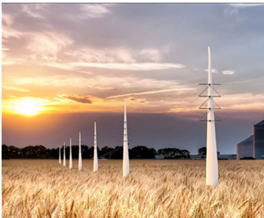
Figure 5. Rendered Wind turbine blade utility transmission poles to be constructed in Kansas, USA [34] , Photo credit: Re-Wind Network [32] .
