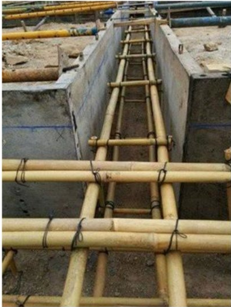
Figure 4. Bamboo in replacement for steel reinforcement.
