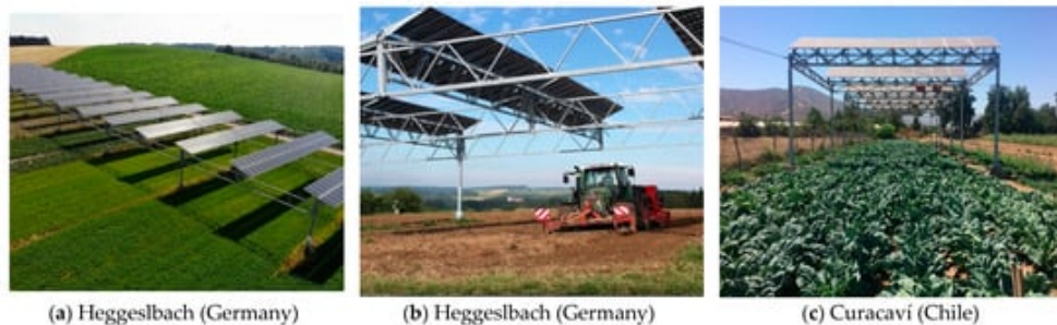
Figure 2. Experimental agrivoltaic systems installed by Fraunhofer ISE in Germany (a,b) and Chile (c). © Fraunhofer ISE.
