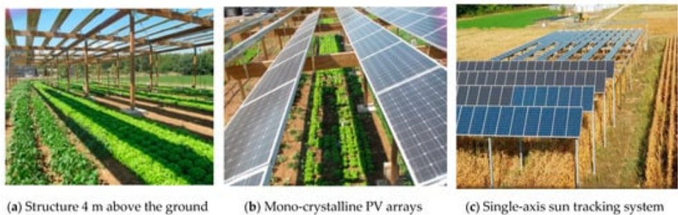
Figure 1. Experimental agrivoltaic system in Montpellier, France. © C. Dupraz.
