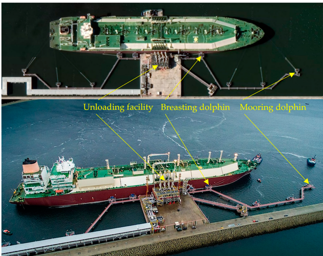
Figure 2. Unloading jetty and LNG carrier (based on [7]).
