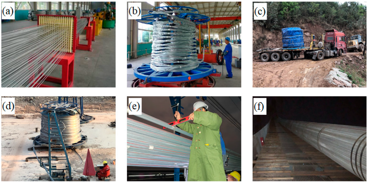
Figure 2. The main procedures of the PPWS method: (a) arrangement and binding of the steel wire, (b) the strand forming, (c) transportation of the strand, (d) the traction of the strand, (e) adjustment of the strand, (f) main cable forming.
