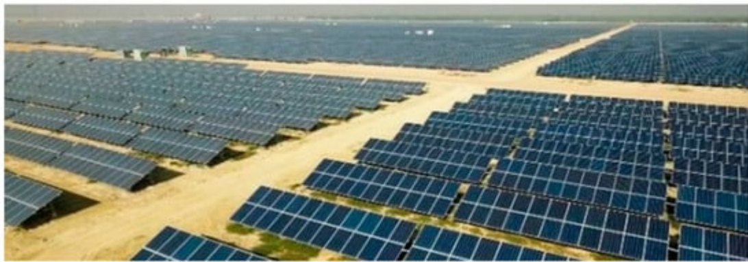
Figure 9. Quaid-e-Azam Solar Park in Pakistan [19] .
