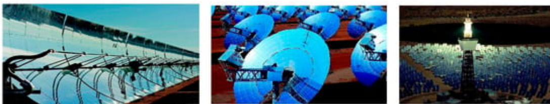
Figure 5. Various solar thermal energy collectors with concentrating mirrors [13][14].
